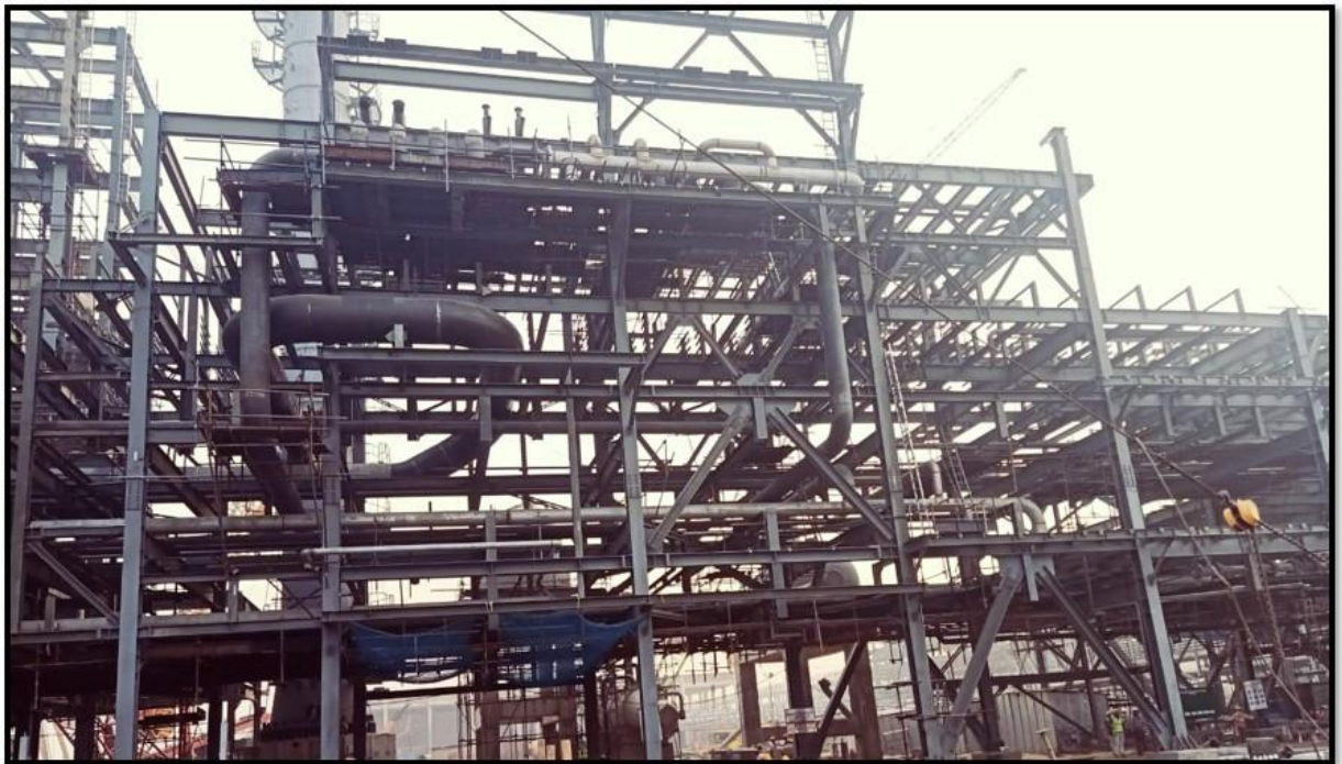
HURL-Barauni-Urea Piping Errection
