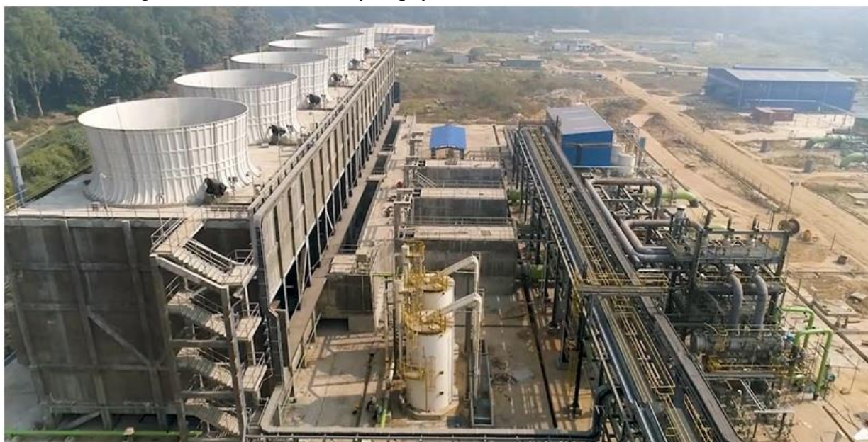
HURL-Gorakhpur-Urea Cooling Tower
