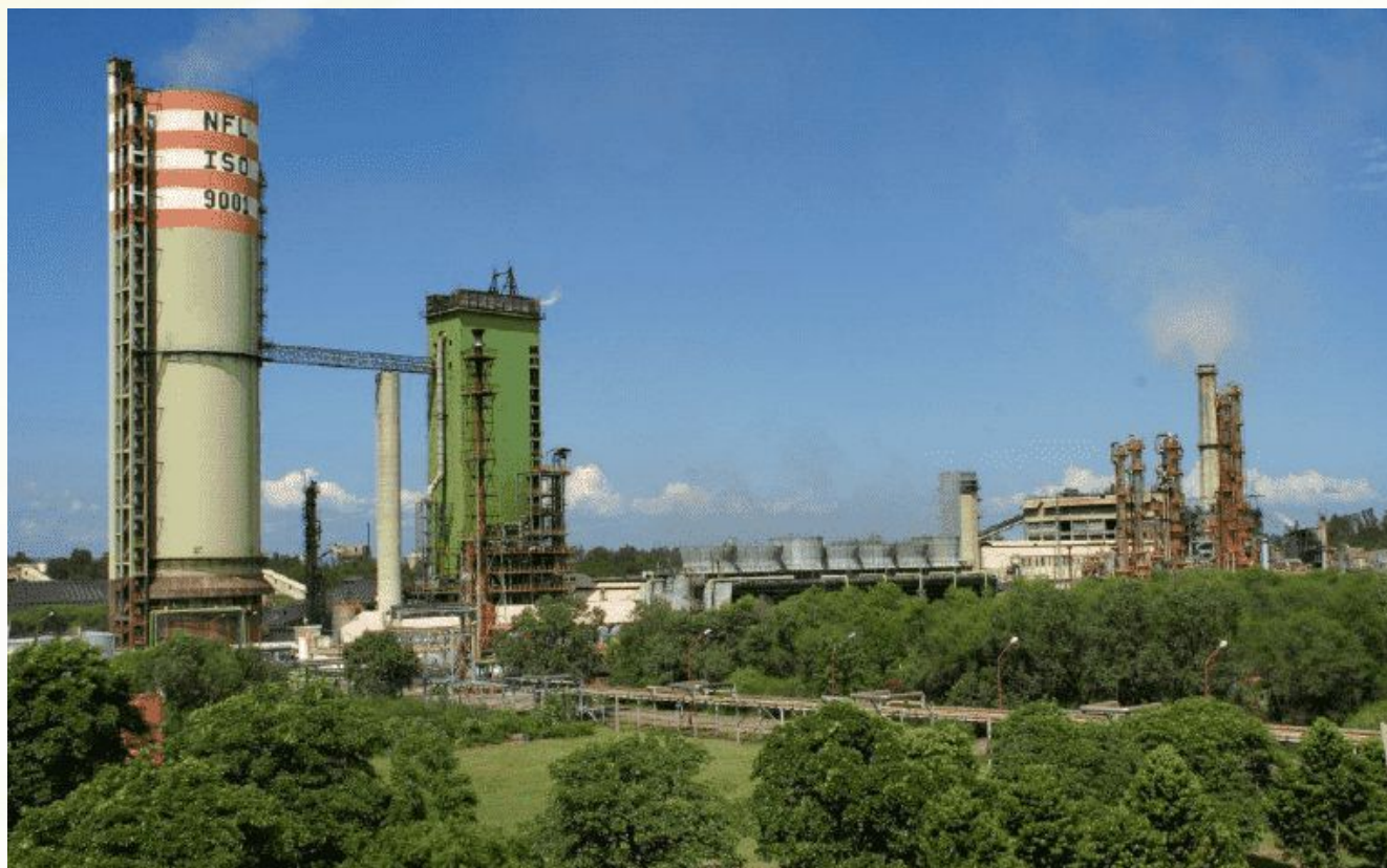
NFL NANGAL PLANT
